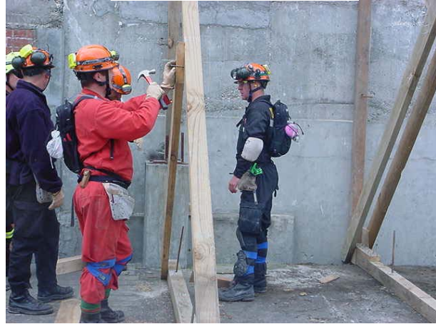
Above: NZ Task Force Technicians practice their shoring techniques.
